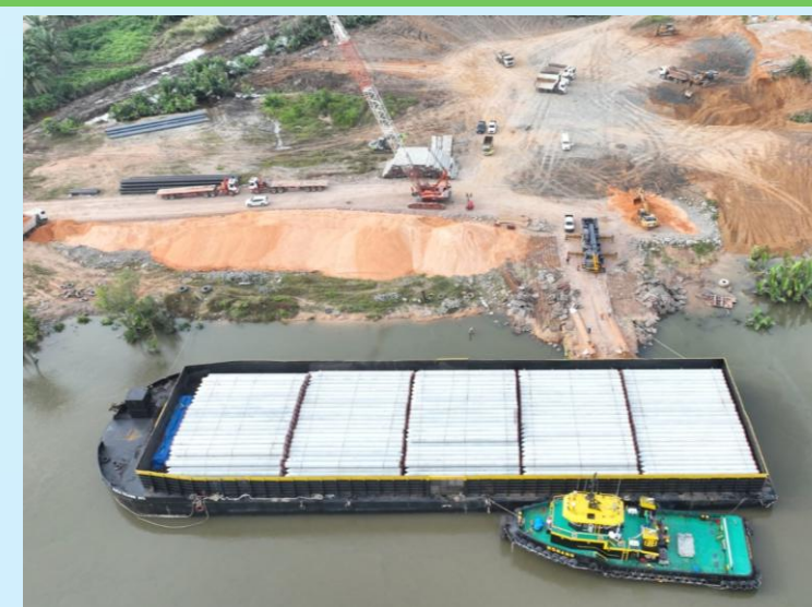
Shoring Protection Area Shiploader Tanah Grogot, Kalimantan Timur
